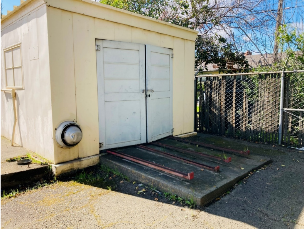
Chlorination facility, view from the driveway off Northgate Blvd
