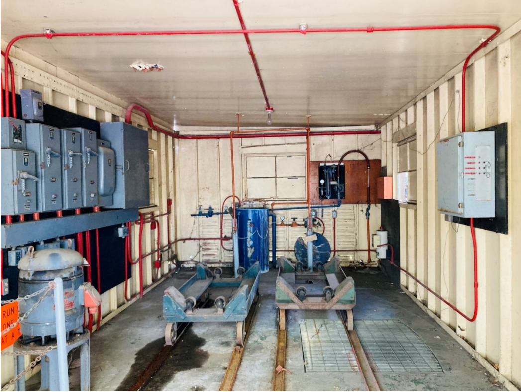
Interior of the chlorination structure, view from the door
